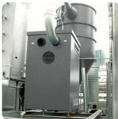
Filtration unit with explosion protection
