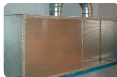
Extraction wall with perforated metal insert
