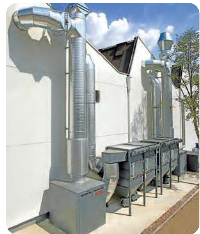
Central extraction systems with two DUSTMAC S filter modules each
